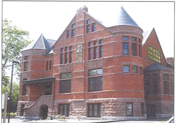
The outside of Senior Living at Prouty shows little of the amount of work that was done inside to create three dozen apartments for low-income senior citizens.
